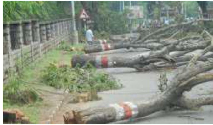
Plate 7. Cutting Avenue Trees for Road Widening in Krishnaraja Sagar Road
