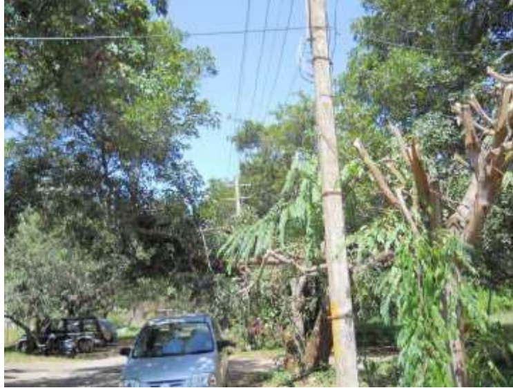
Plate 3. Avenue Trees are chopped by Electricity gang men clearing the way for overhead lines - Manasagangotri Campus
